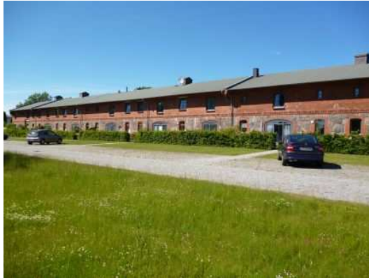
Fig. 5: For living purposes redesigned farm buildings on the domain of Ferdinandshof near Pasewalk.
